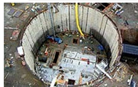
Eastside Combined Sewer Overflow Tunnel Boring Project – Portland, Oregon, USA
